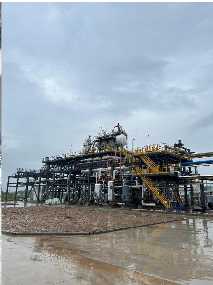
Figure 3: Super Claus furnace used at the insoluble sulphur production line to reduce emissions and recycle sulphur. According to Sunshine, the group is the first company in China to invest in a Super Claus furnace
